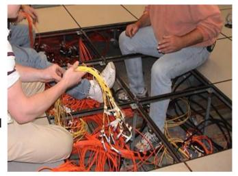
Having a crawl space allows networking cables, electric wiring, and water pipes to be placed under the equipment they support for more efficient connectivity, power or cooling. Because all of the cables, wires and pipes are out of the way, using the crawl space also eliminates safety hazards on the raised floor itself.
